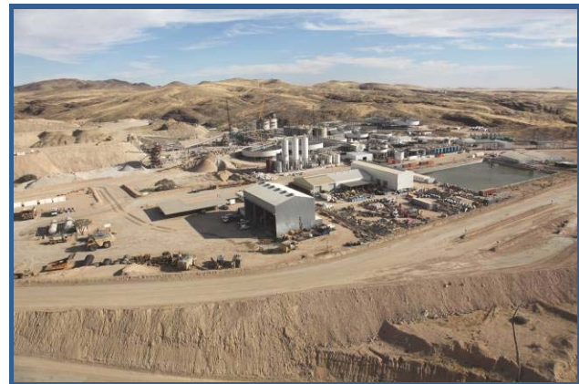
OVERALL PLANT VIEW
