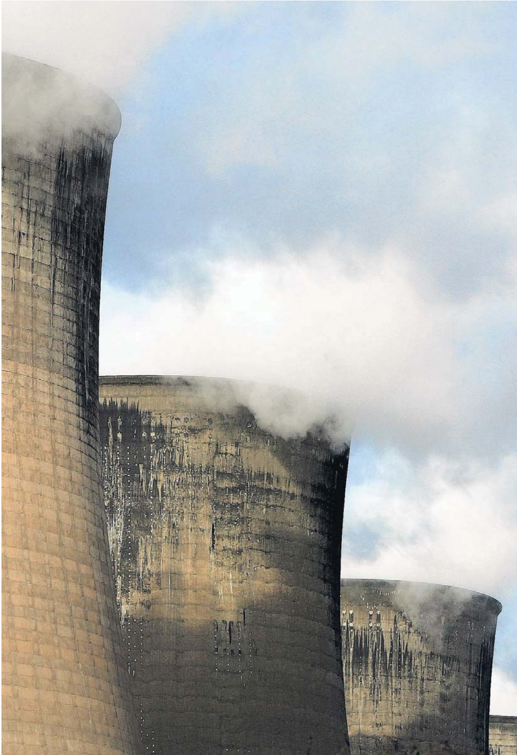
Steam rises from the cooling towers of a coal-fired power station in England. However, China and the US are committed to reducing their carbon emissions. Picture: Getty Images
